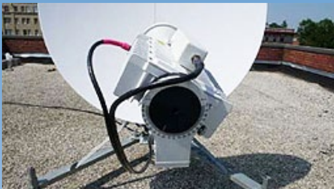
Figure 4: Linear polarization is adjusted by physically rotating the feed assembly
