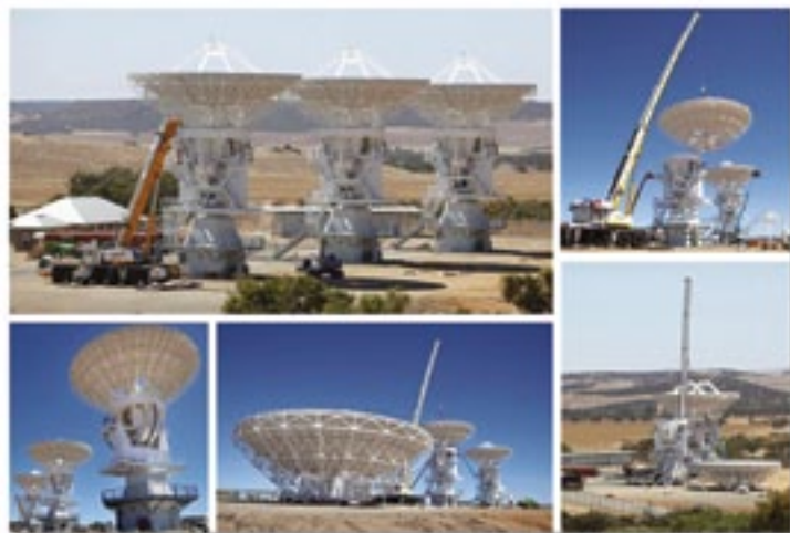
Figure 6. The three Ka-band antennas being installed at the RAF in Geraldton, Australia.
