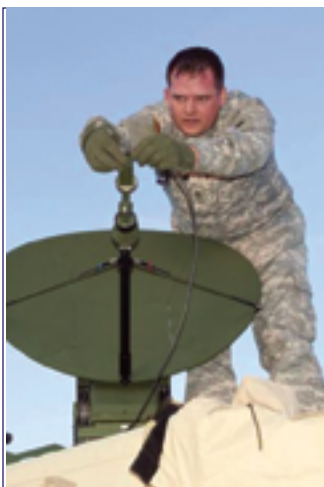
Staff Sgt. Jonathan Means sets up a dish antenna for a satellite unit nicknamed the "Cheetah" as part of a communication exercise for the 63rd Theater Aviation Brigade's signal section in Pensacola, Florida. The Cheetah system is an auto-acquiring portable satellite receiver that provides high-speed data communications for Internet and phone connections in remote locations or following a catastrophic event.
